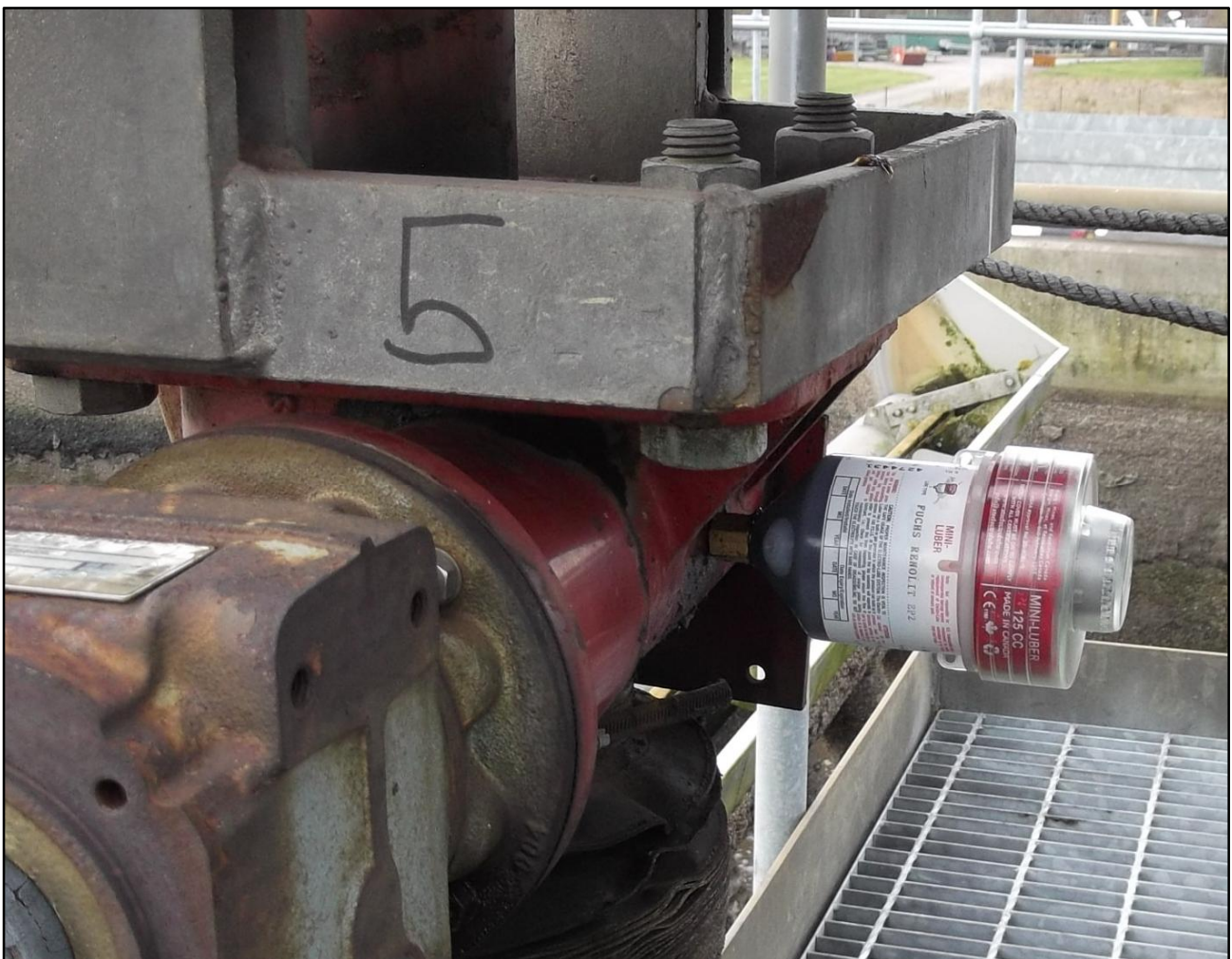
125cc Mini-Luber fitted to Aerator Decanter
