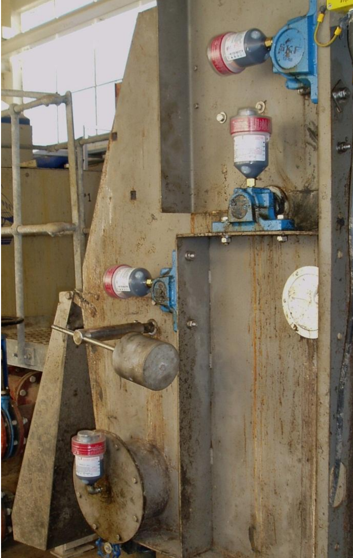
125cc Mini-Lubers fitted to Gravity Belt Thickeners
